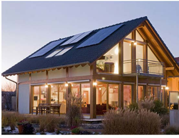
Home photovoltaic system
